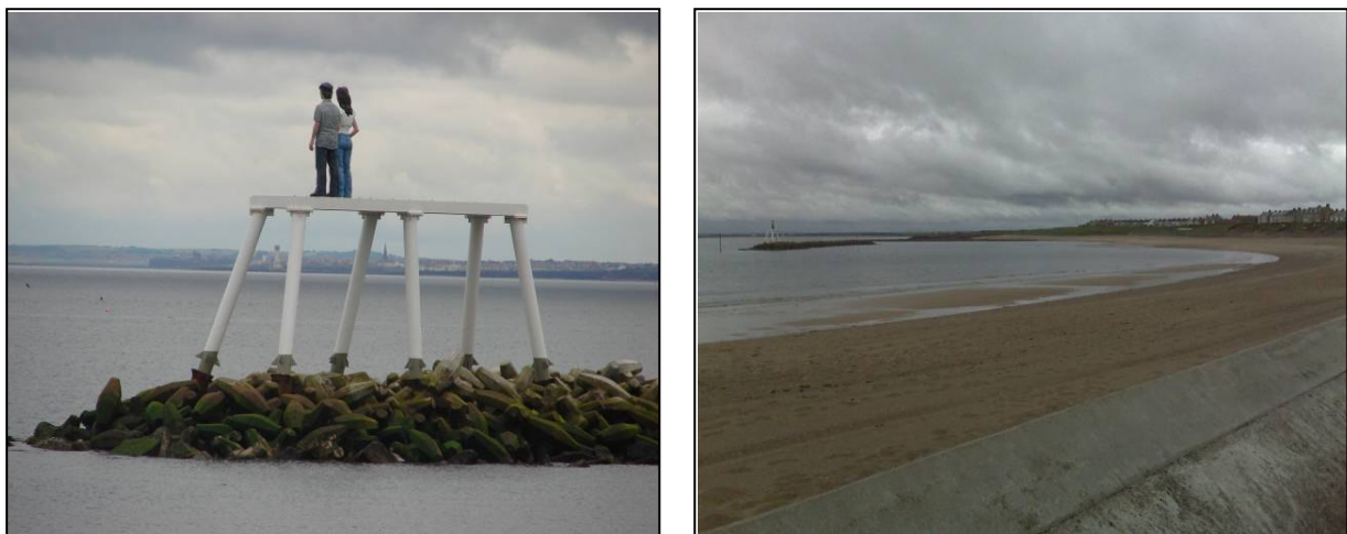
Figure 7. Newbiggin Bay Coast Protection Scheme: Offshore Breakwater (left) and Replenished Beach (right)
