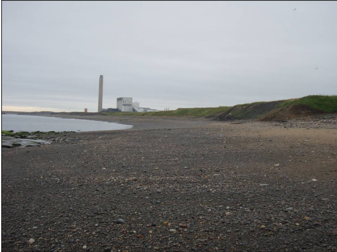
Figure 4. Slag Bank in northern Lynemouth Bay located high up the beach profile
